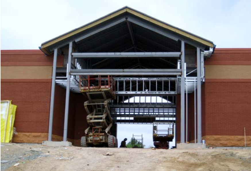
Framing at front entrance to the building
