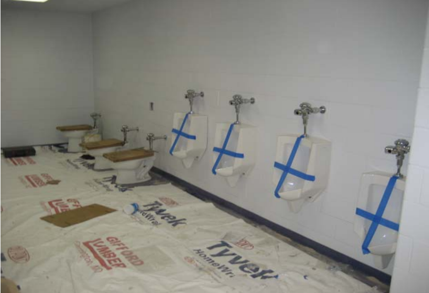
Restrooms with fixtures installed
