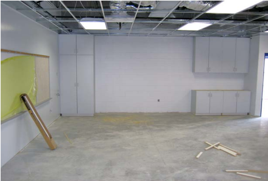
Typical classroom marker/tack boards and cabinetry installed
