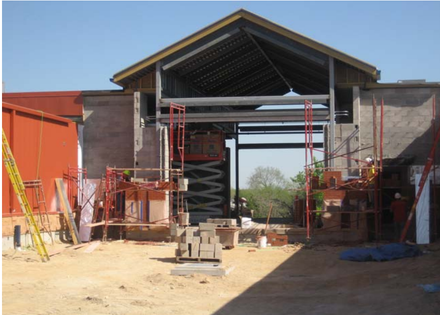
Lobby courtyard side work on masonry columns
