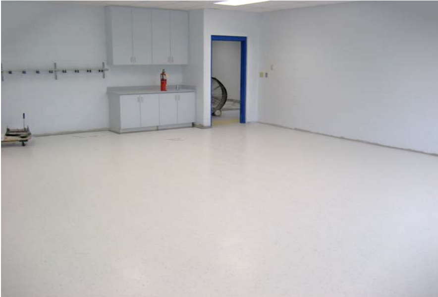
Typical classroom with VCT installed
