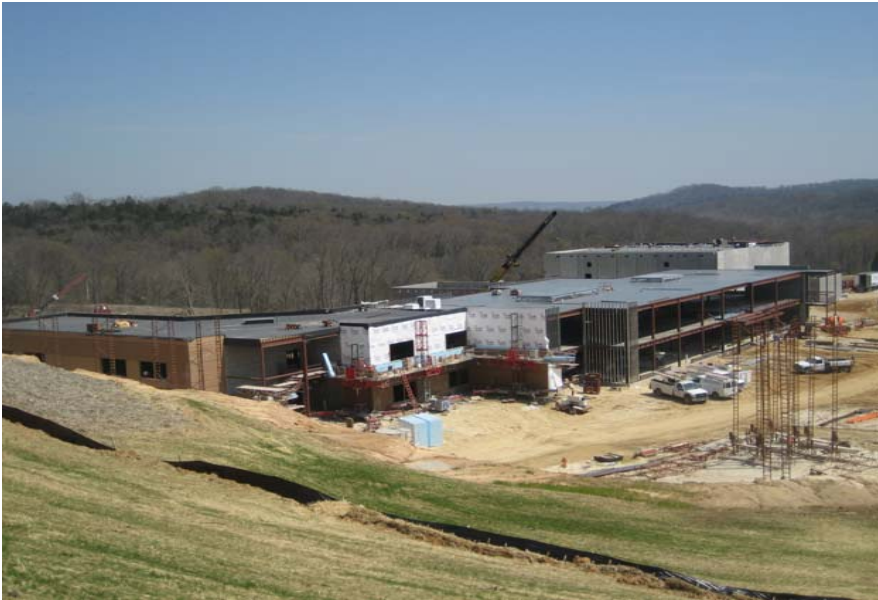
Mid April 2009 building progress
