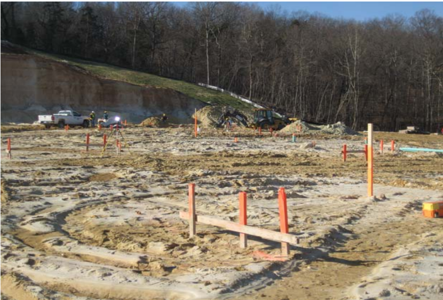
January 2, 2009 - Goodwin Brothers Began Layout of Footings
