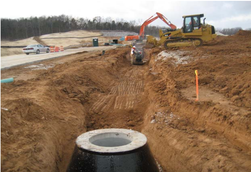
December 1, 2008 - Site Utility Contract Work Begins
