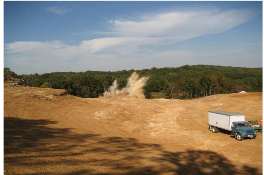
October 10, 2008 - Blasting Rock
