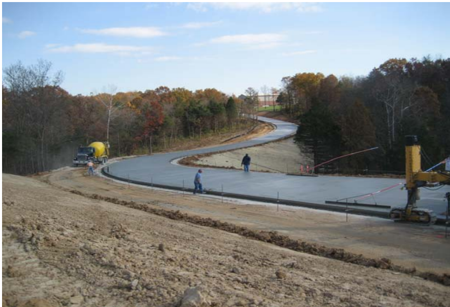
November 3, 2008 - Main Entrance Roadway Paved
