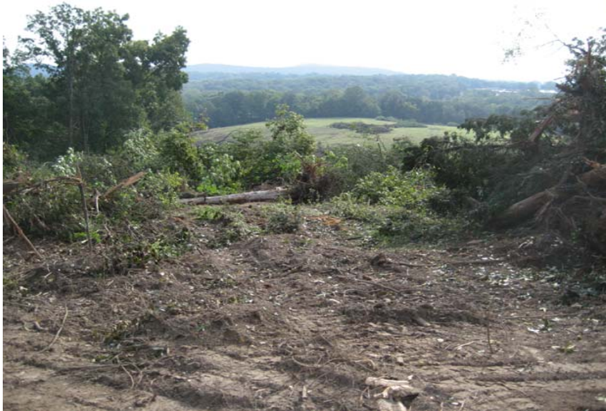
September 18, 2008 - Site Clearing Began
