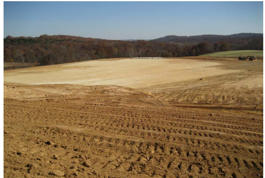
November 7, 2008 - Site Grading Package Completed; Building Pad Ready
