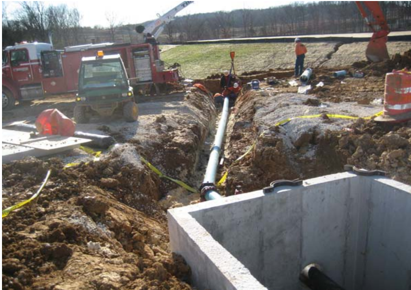
Installation of 12 x 8 tee to the meter pit
