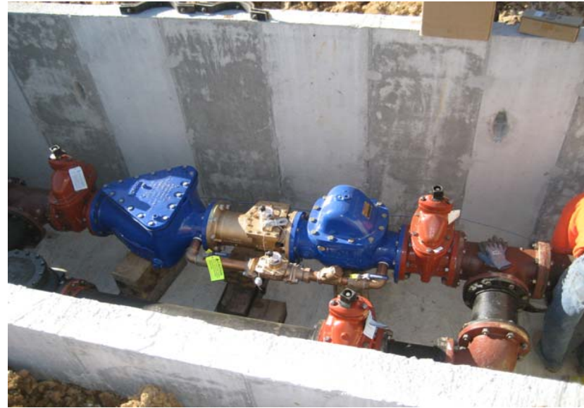
The meter pit with valve and piping installed
