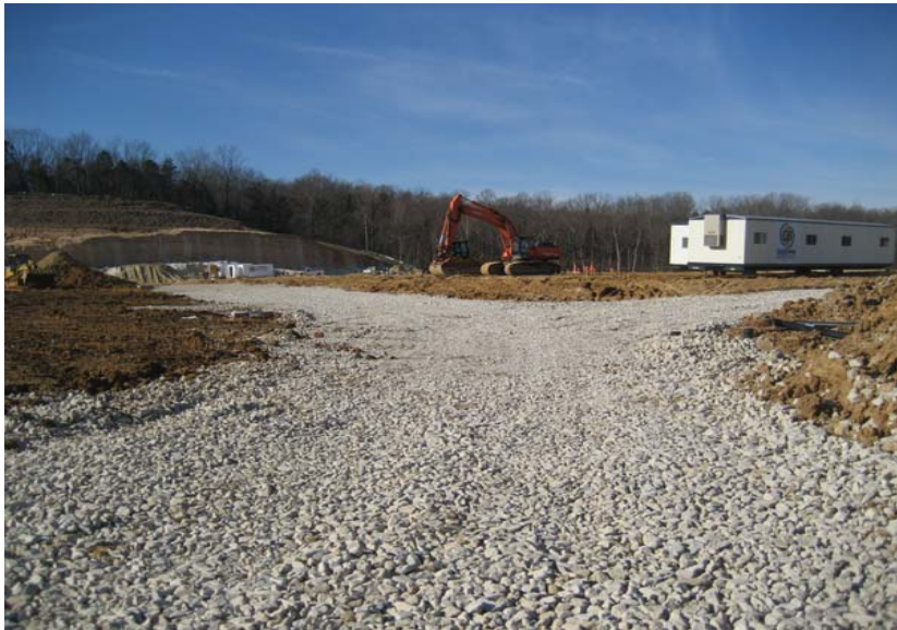
Rocked roadway provides access to the jobsite
