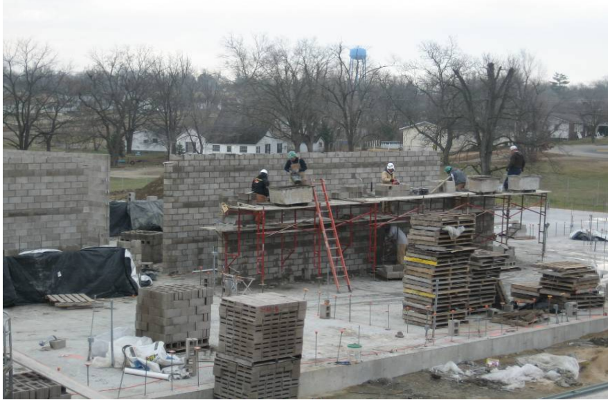
Progress on classroom wing load bearing walls
