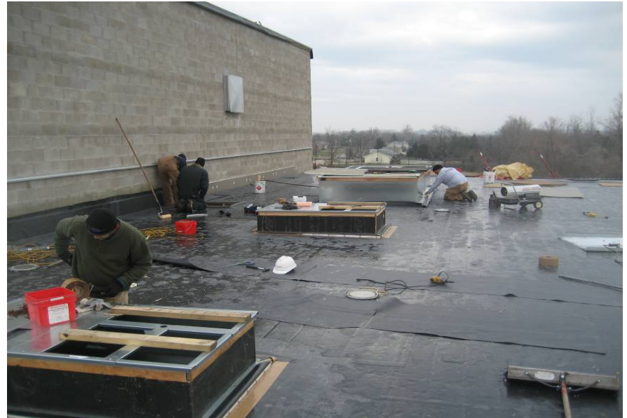
Installing roofing over gym classroom area
