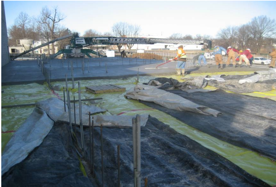
Pouring Fine Arts area slab. Blankets are removed as pour progressed
