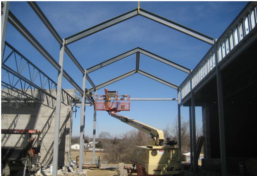
February 26 - Fine Arts section joist set; working on lobby steel
