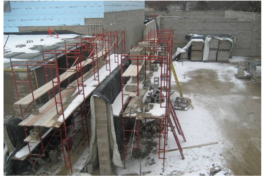
February 12 - Jobsite covered with snow and ice
