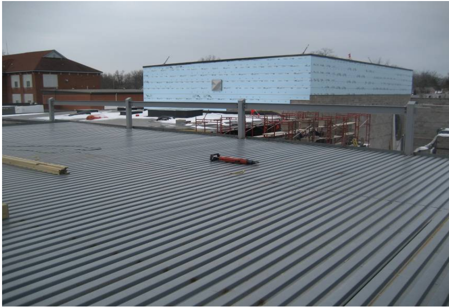
February 12 - Work on lobby steel to complete Office/Admin roof deck
