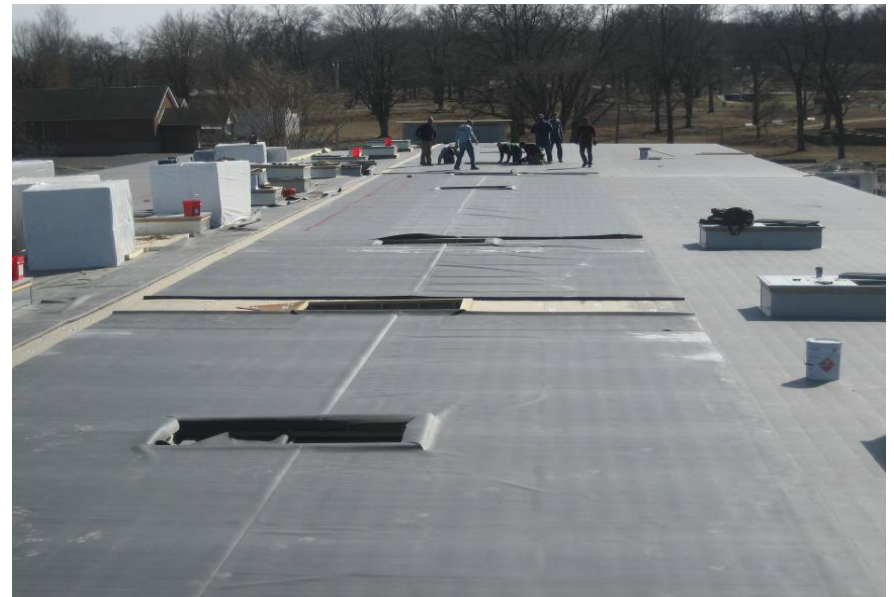
February 26 - Classroom wing roofing about 90% complete
