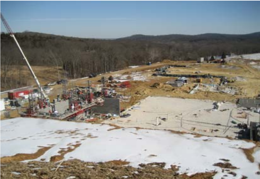
North Portion of the Building Site February 6th Progress
