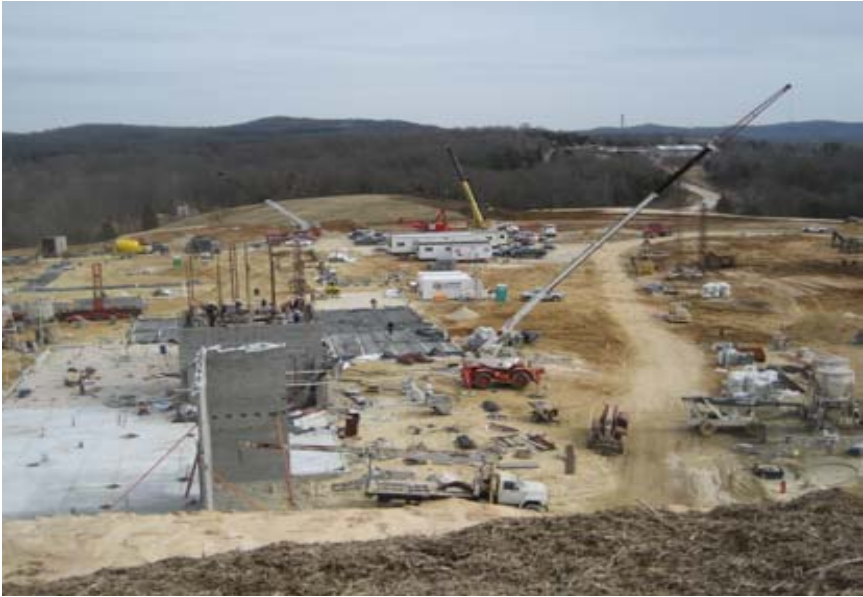
South Portion of the Building Site February 20th Progress
