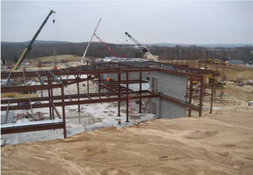
South Portion of the Building Site February 27th Progress
