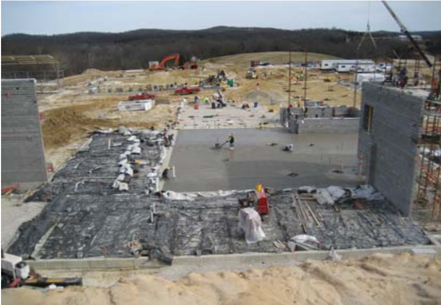
South Portion of the Building Site February 13th Progress
