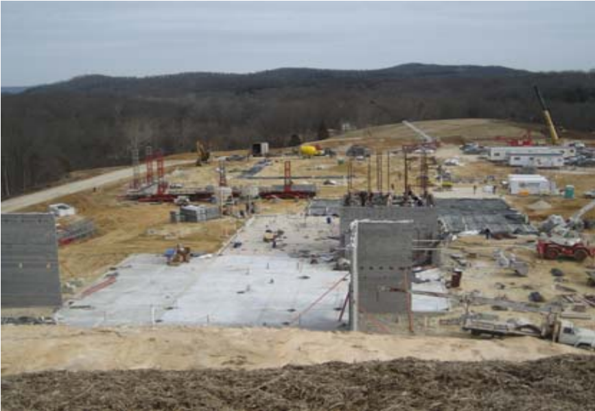
North Portion of the Building Site February 20th Progress
