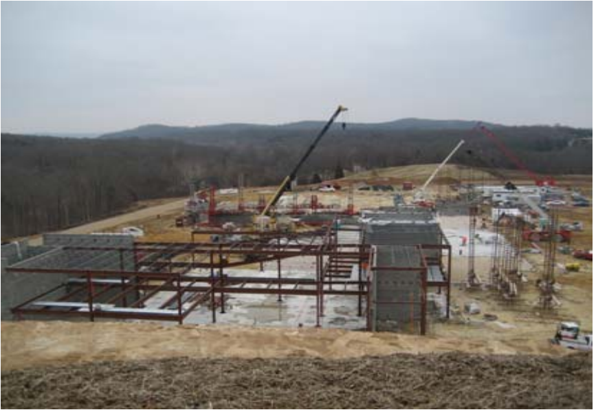
North Portion of the Building Site February 27th Progress
