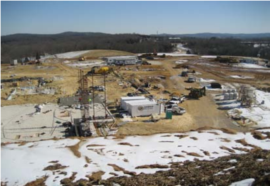
South Portion of the Building Site February 6th Progress
