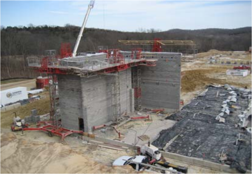
North Portion of the Building Site February 13th Progress
