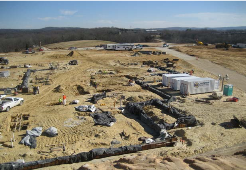
Progress on Building south side - January 22, 2009
