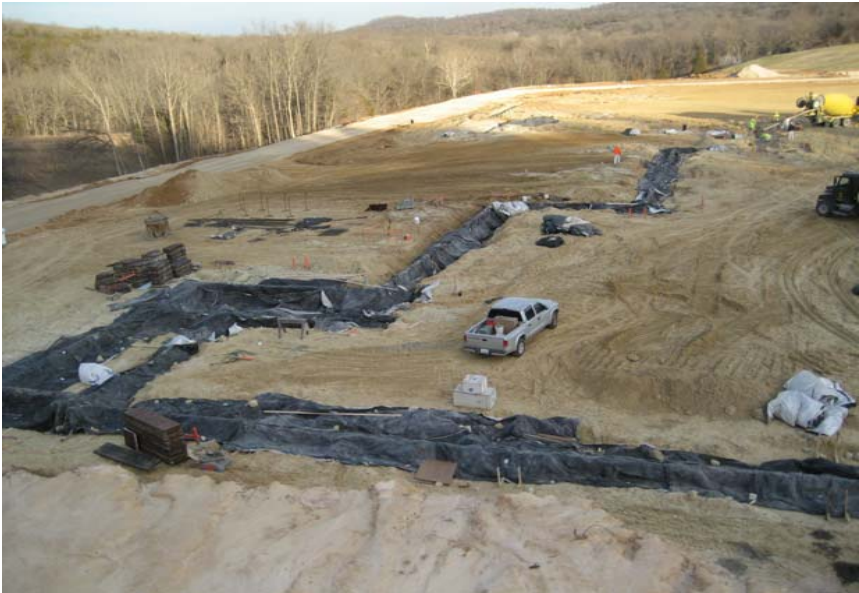
Progress on Building north side - January 9, 2009
