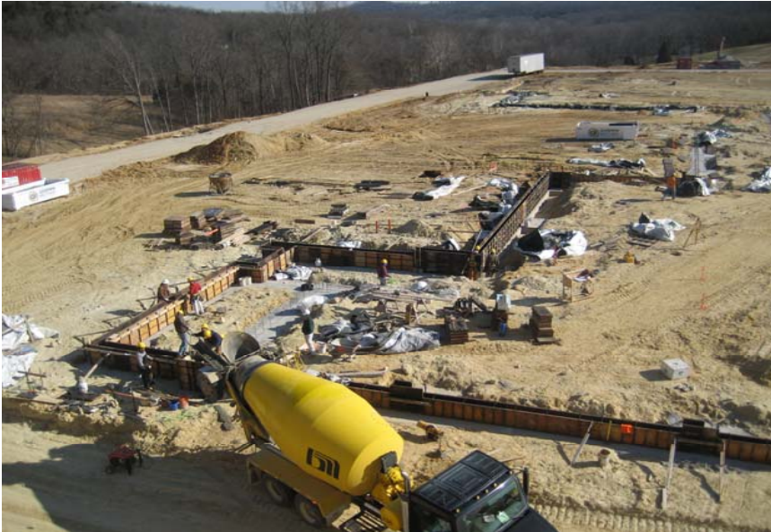
Progress on Building north side - January 17, 2009
