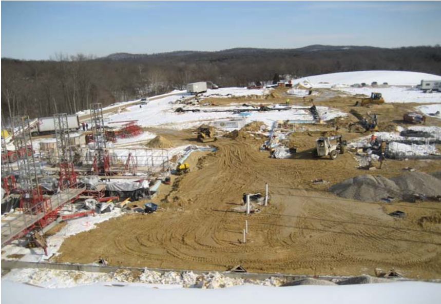
Progress on Building north side - January 30, 2009
