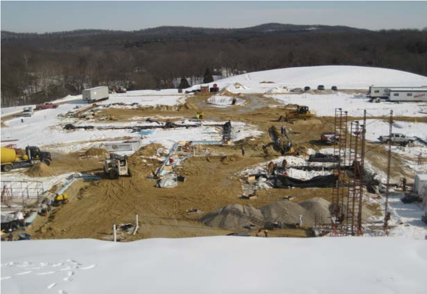
Progress on Building south side - January 30, 2009
