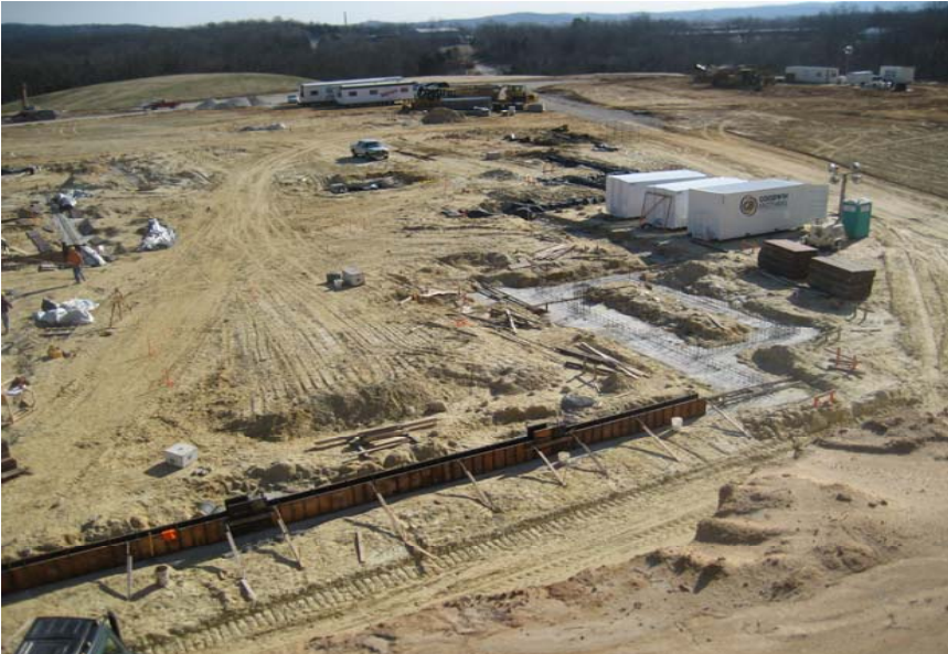
Progress on Building south side - January 17, 2009
