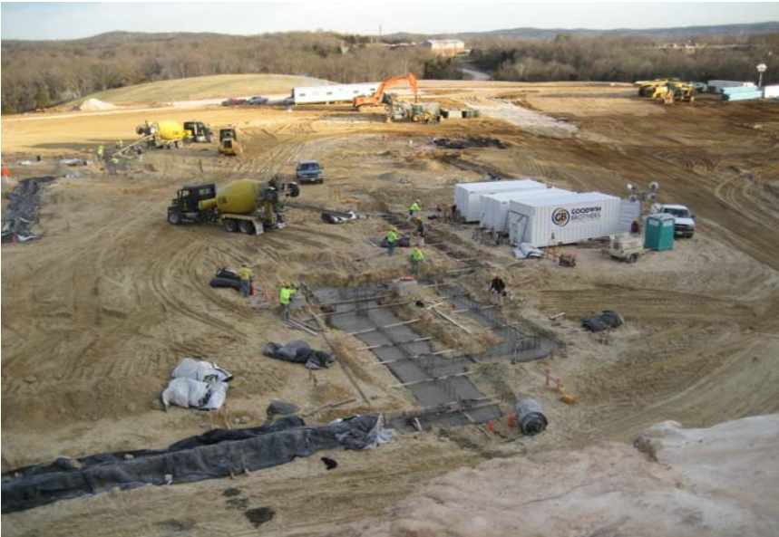
Progress on Building south side - January 9, 2009
