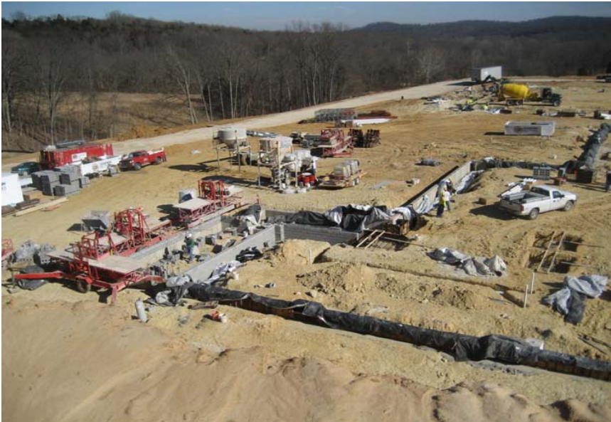
Progress on Building north side - January 22, 2009
