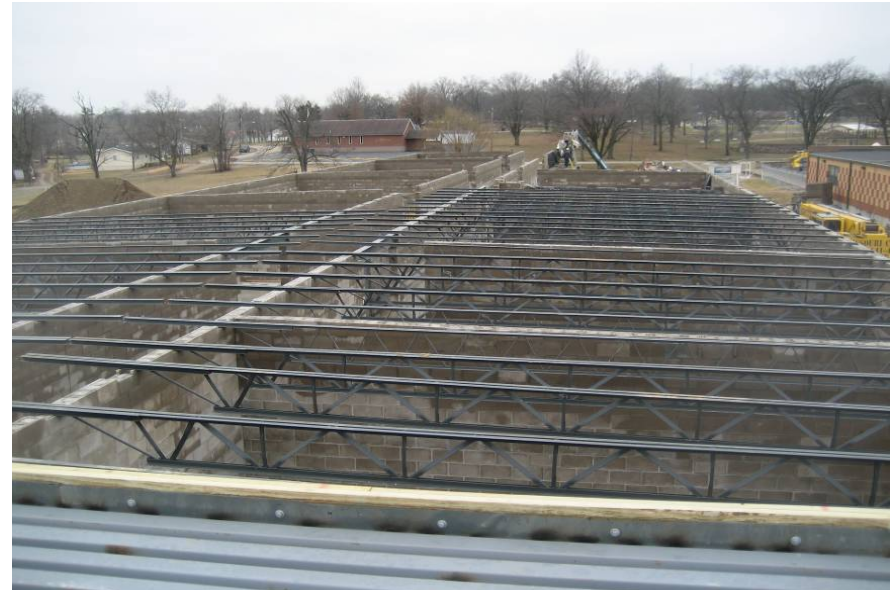
January 22 - Joist set over north 2/3rd of classroom wing
