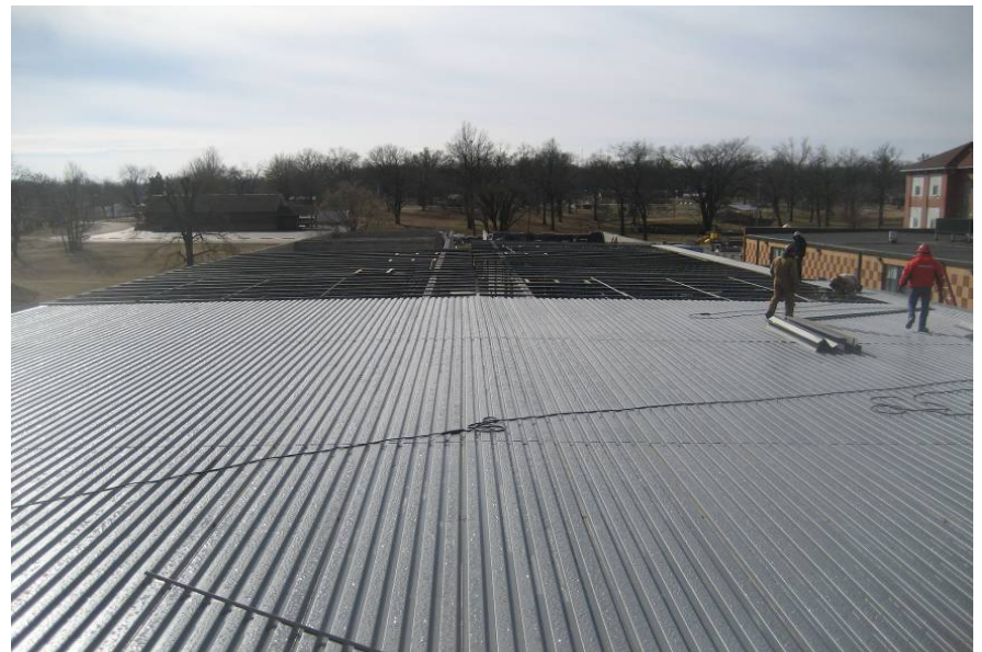
January 28 - Progress on welding joist and deck over classroom wing
