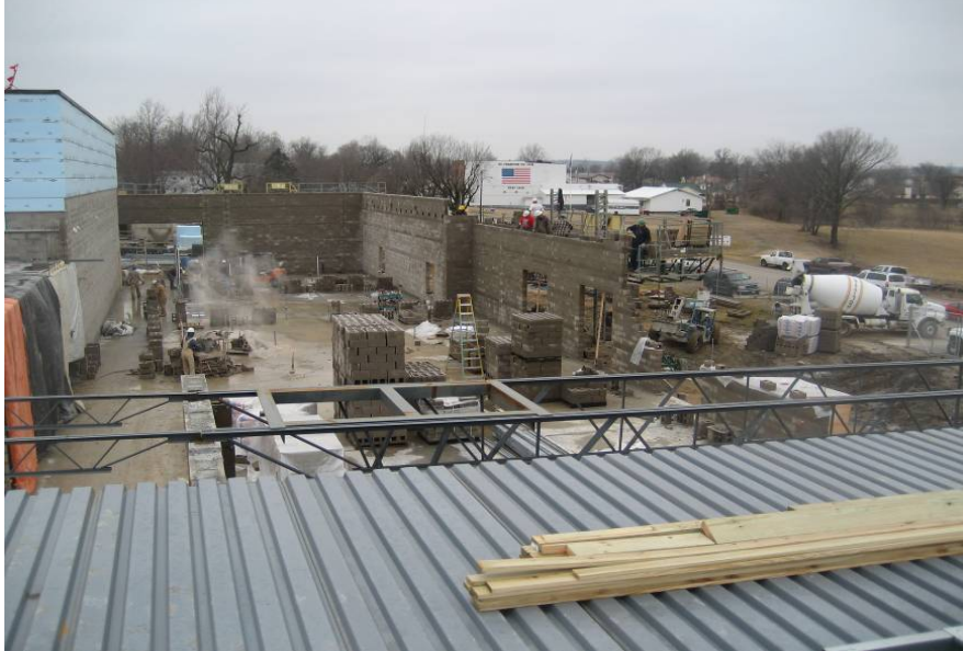
January 22 - Progress on CMU walls in the fine arts area
