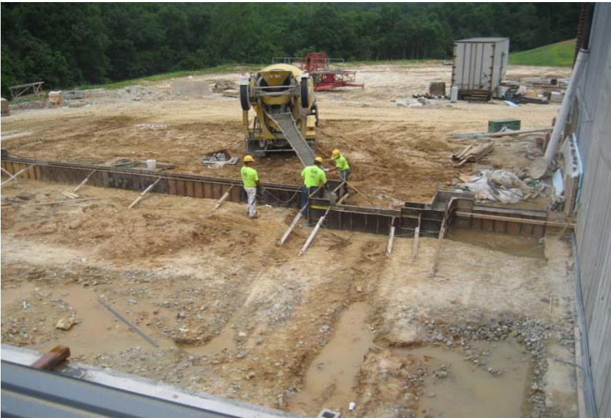
June 12, 2009 - Weight room foundation walls are poured
