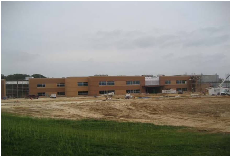
June 12, 2009 - Progress on south building elevation
