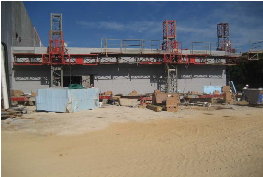
June 30, 2009 - Weight room load bearing walls completed
