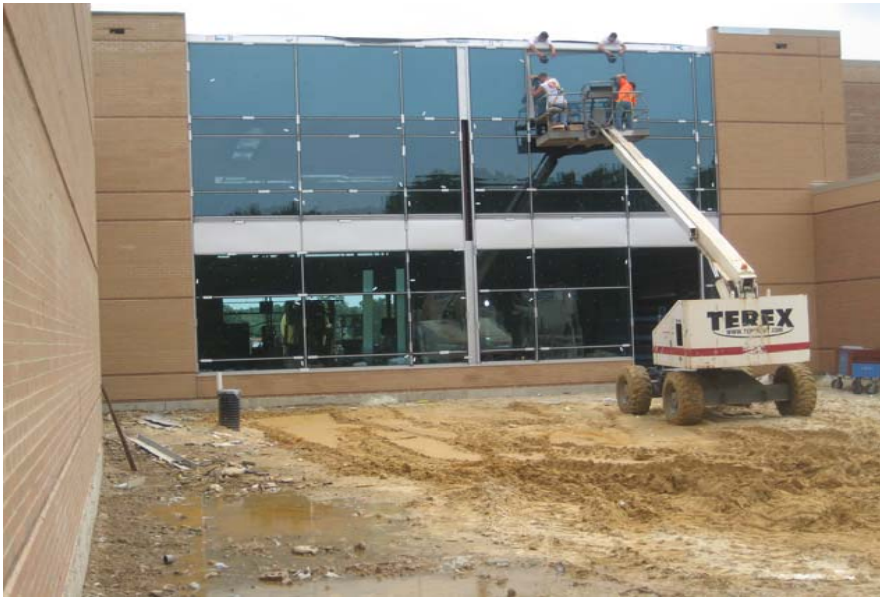
June 12, 2009 - Progress on north building elevations
