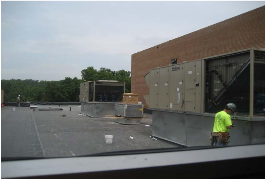
June 2009 - The gym roof top units are set
