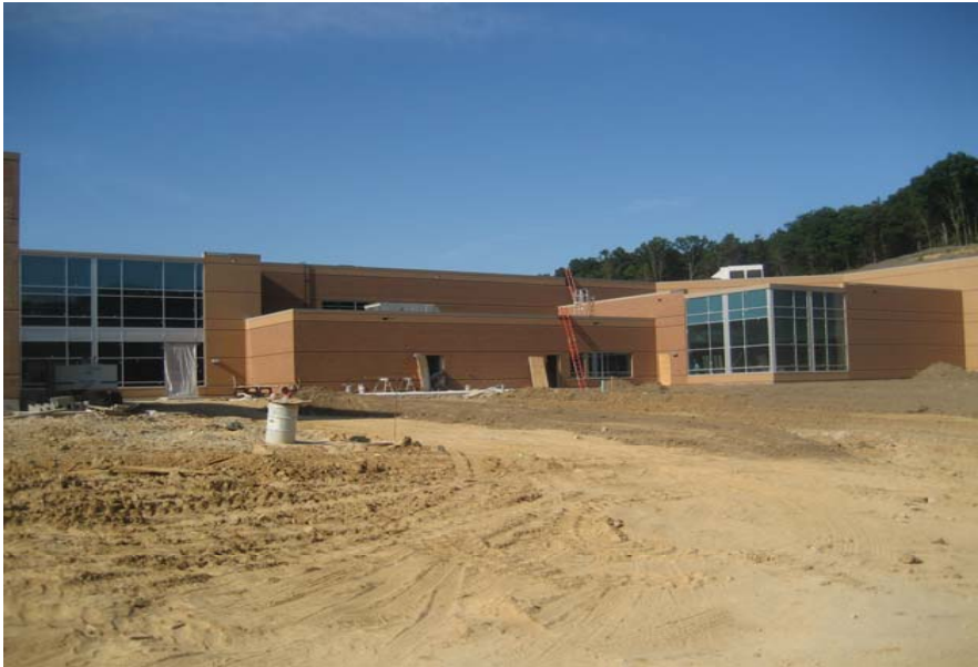
June 30, 2009 - North elevation of the building
