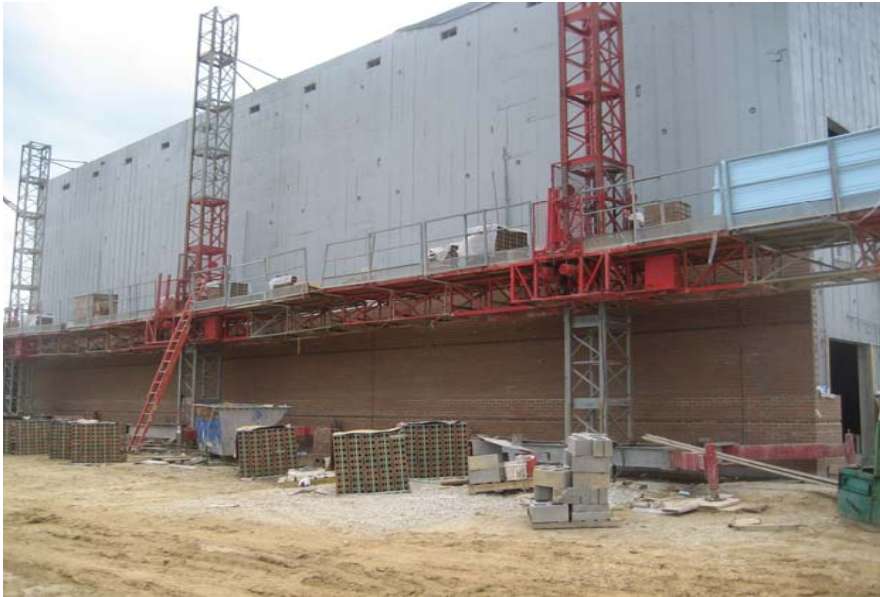
June 2009 - Brick veneer work on the east elevation of gym
