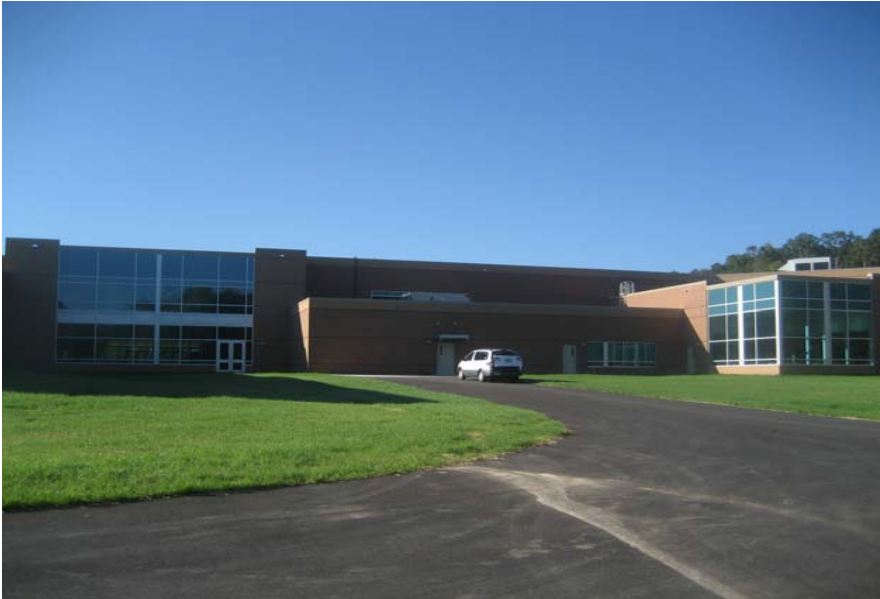
Rear elevation of A-building; glass planted and growing.
