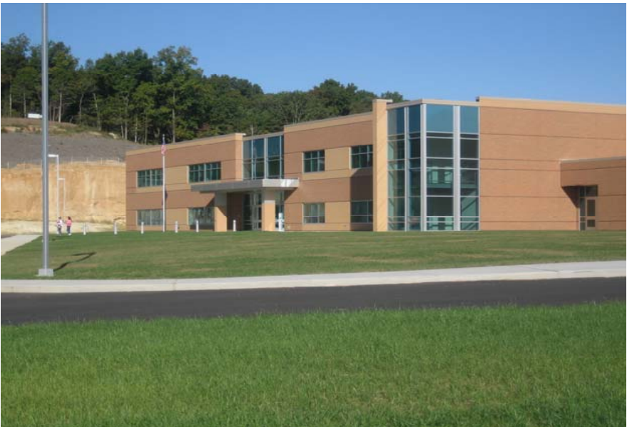
Front elevation and entry A-building with lawns in place.
