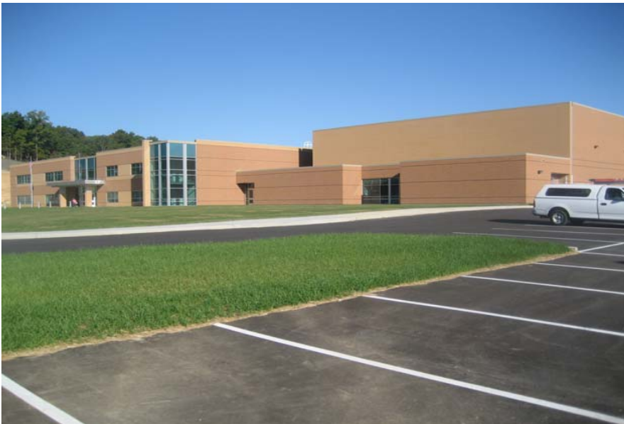
Front elevation of B-building with lawns in place.
