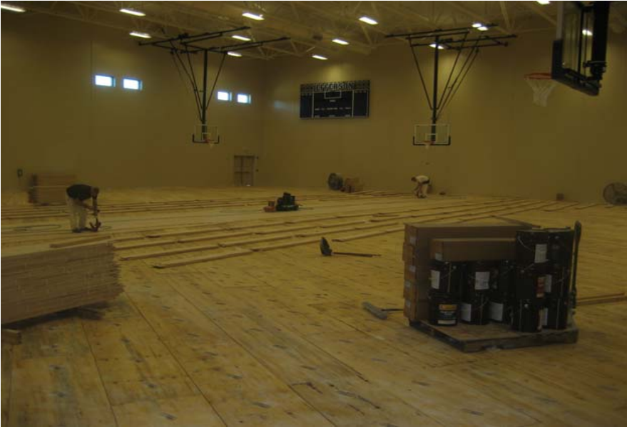
Wood floor in gym being installed.
