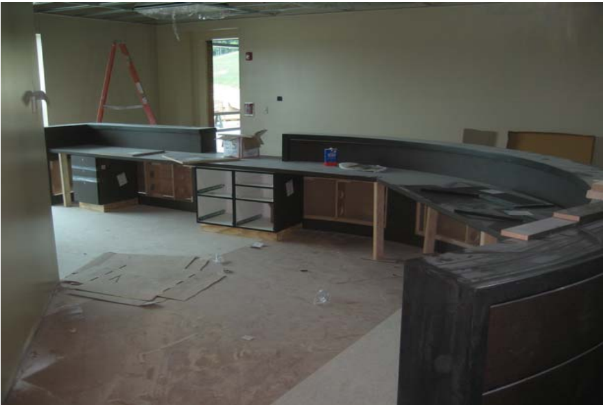
Casework being install in the Administration Reception Area
