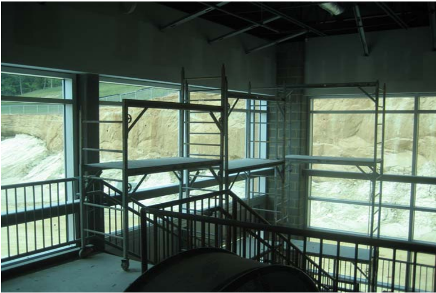
Finishing touches on one of the three stair towers
