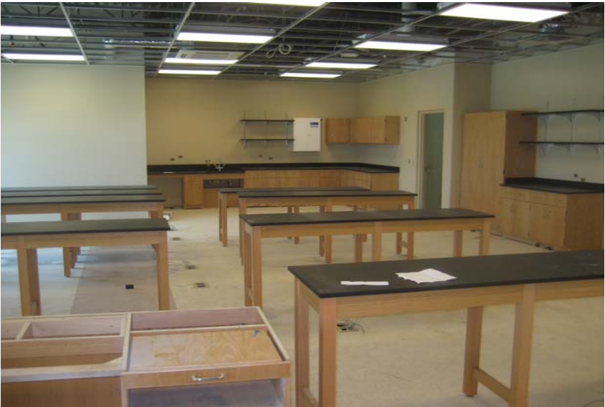
Science Lab casework being installed
