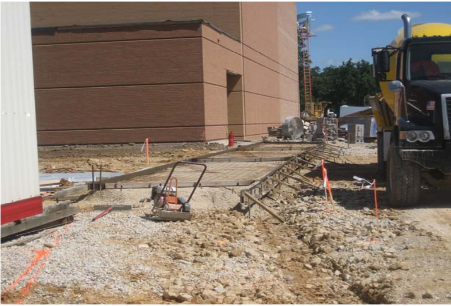
Concrete walks around site being formed and poured
