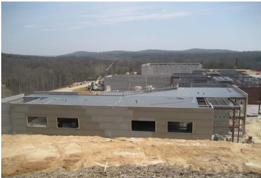
March 27, 2009 - Progress on the north side of the building
