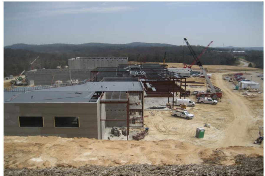
March 27, 2009 - Progress on the south side of the building
