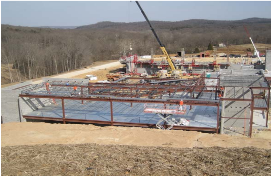
March 6, 2009 - Progress on the north side of the building
