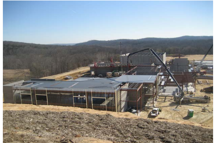
March 20, 2009 - Progress over view of the building
