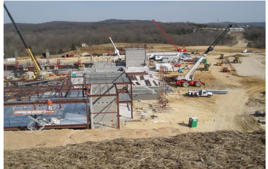
March 6, 2009 - Progress on the south side of the building
