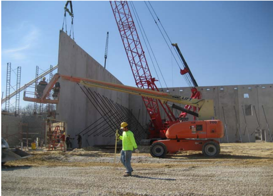
March 13, 2009 - Setting of precast concrete wall panels of the gym
