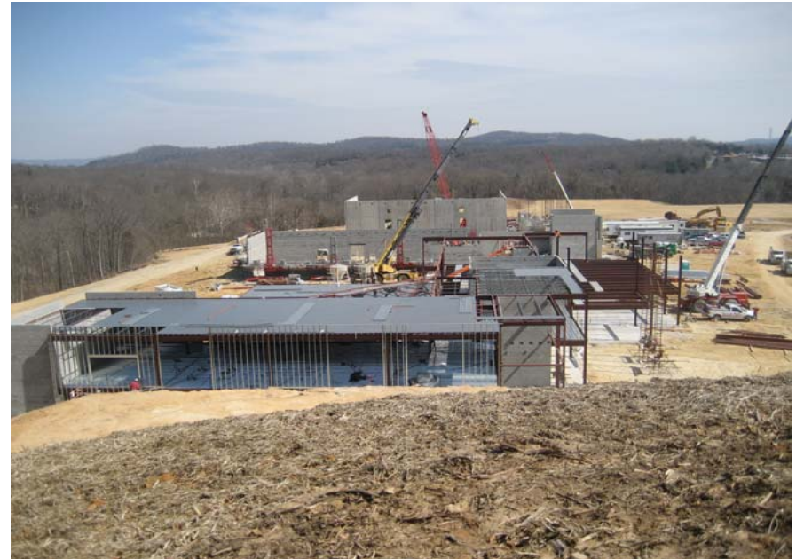
March 13, 2009 - Progress overview of the building
