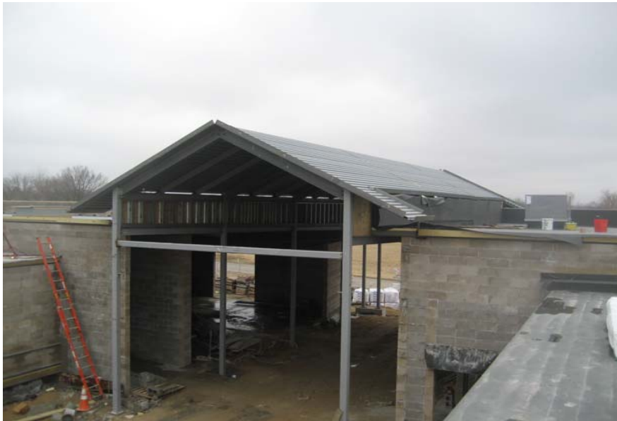
Lobby roof prepped and ready for standing seam roof
