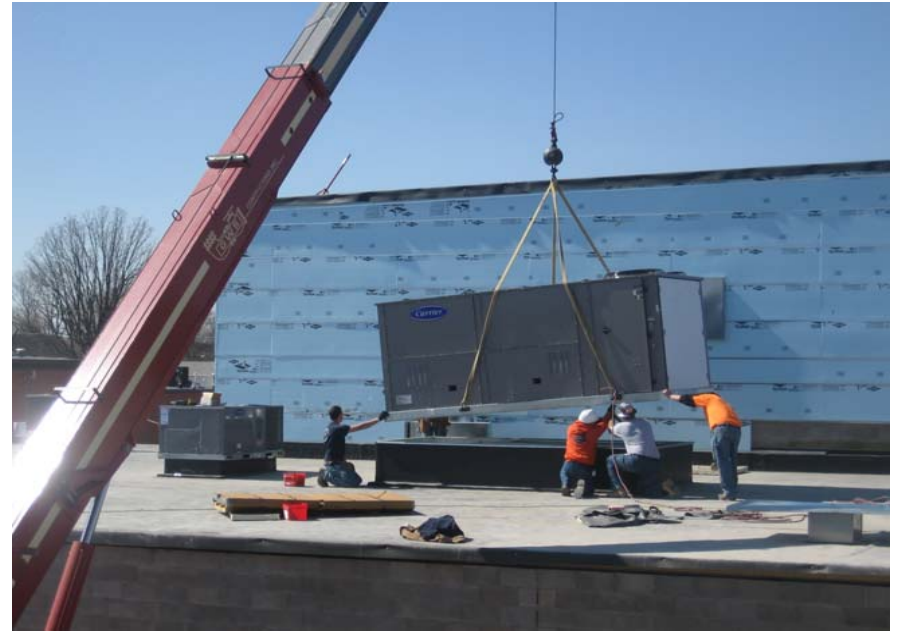
Setting RTUs; this unit serves the gym
