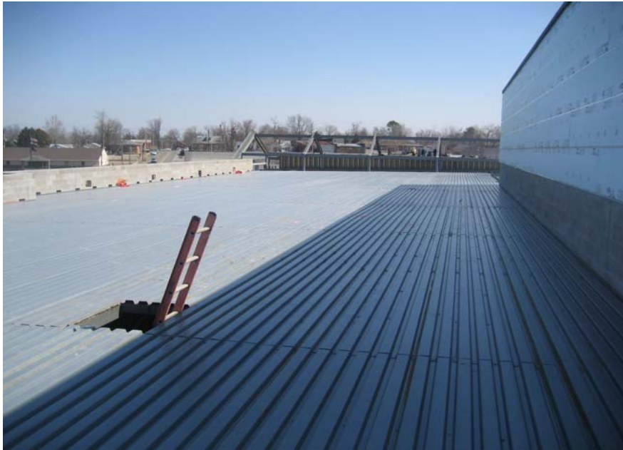
Fine Arts area roof deck installed
