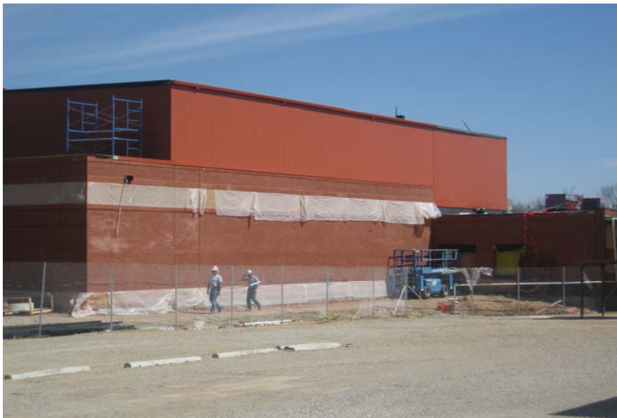
Brick veneer work completed; metal siding and trim installed
