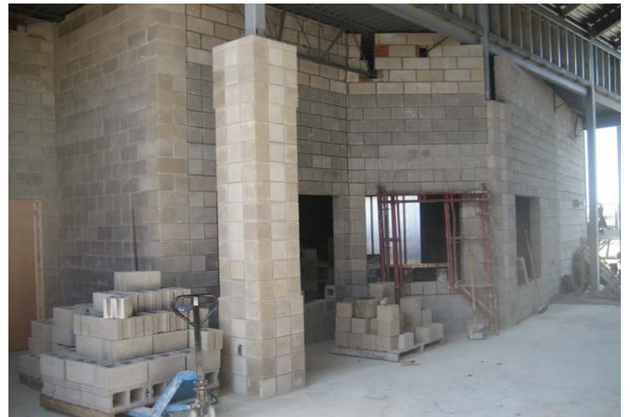
Lobby CMU walls and columns completed
