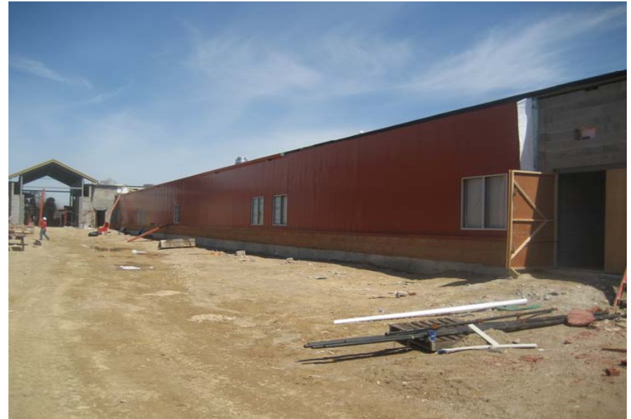
Metal siding installed; stone courses installed; windows in place
