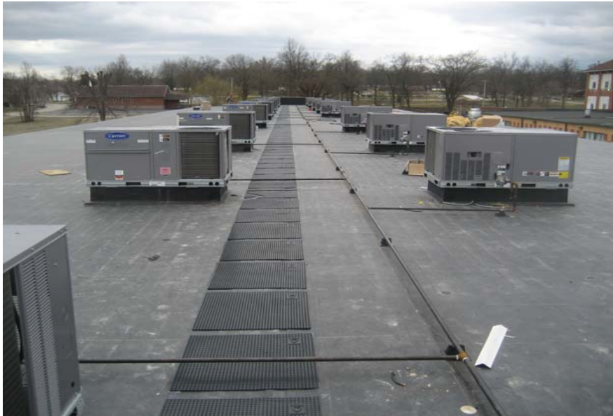
RTUs set; gas piping installed ready to start up
