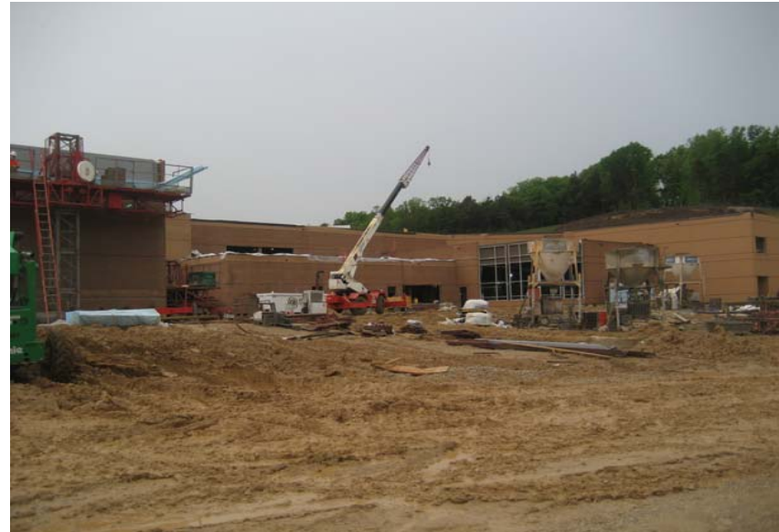
May 8, 2009 - Progress on the north building elevations
