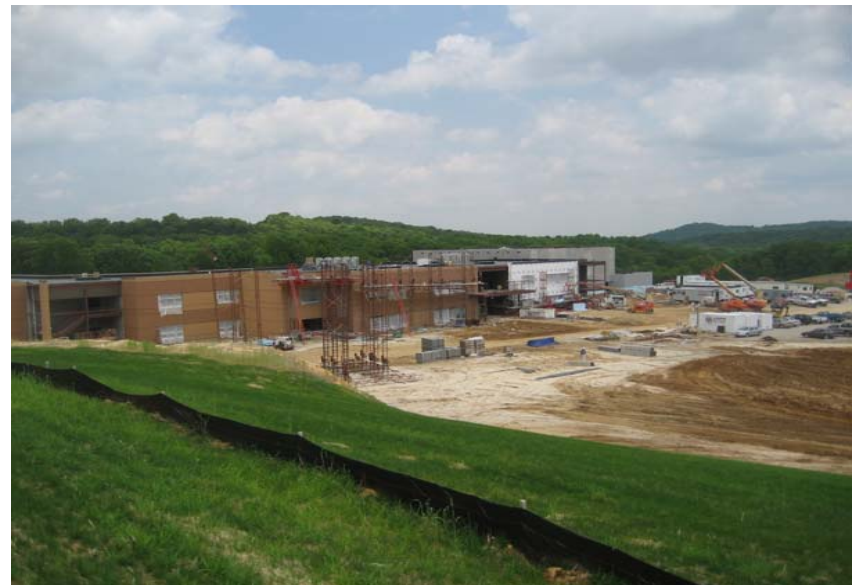
May 15, 2009 - Progress on the south building elevation
