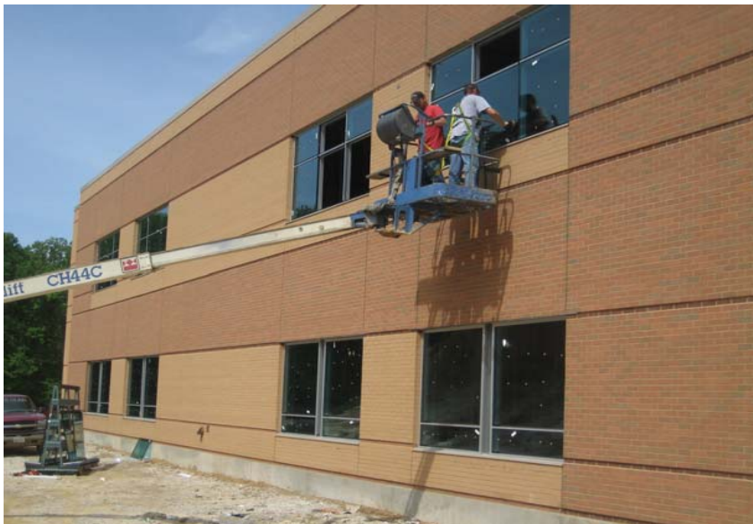
Glazing of window frames on the west building elevation
