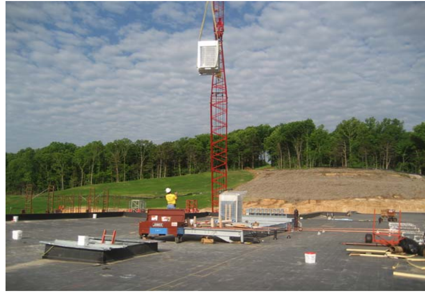
Hoisting of mechanical equipment to roof platforms
