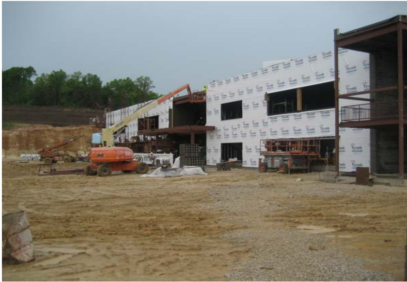
May 8, 2009 - Progress on the south building elevation
