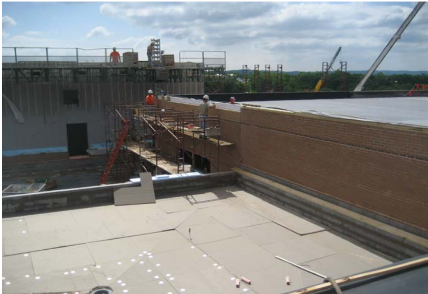
Progress on brick veneer work above roofs over locker rooms
