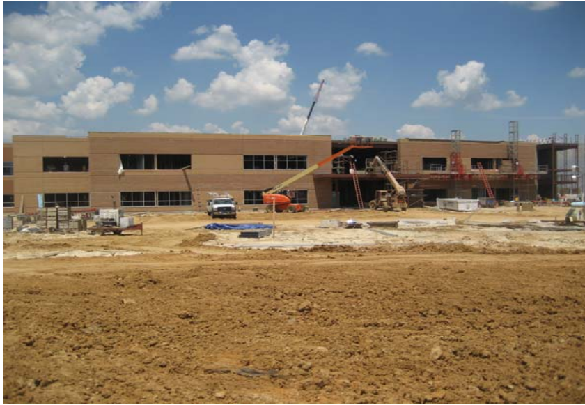
May 22, 2009 - Progress on the south building elevation
