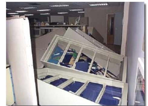
This example of non-structural damage is common after earthquakes of even moderate size - © FEMA File Photo
