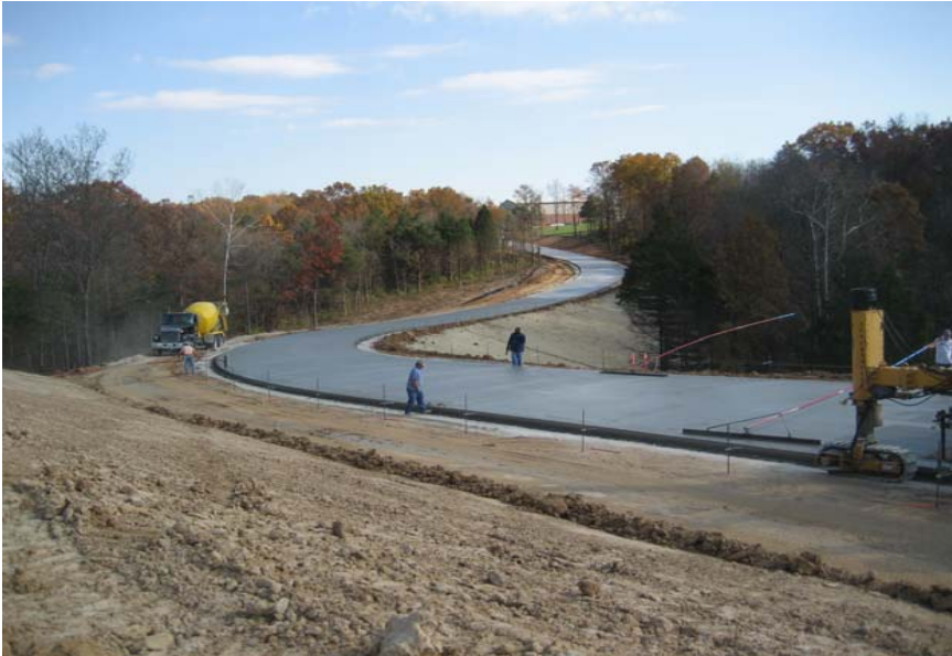
Concrete paving operations approximately 1500 feet from entrance.
