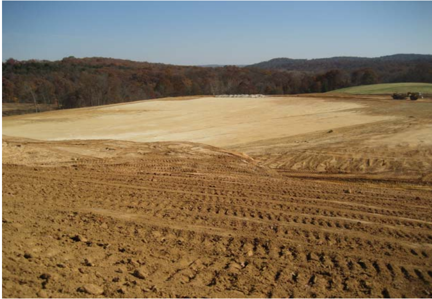
Building pad finished and proof rolled
