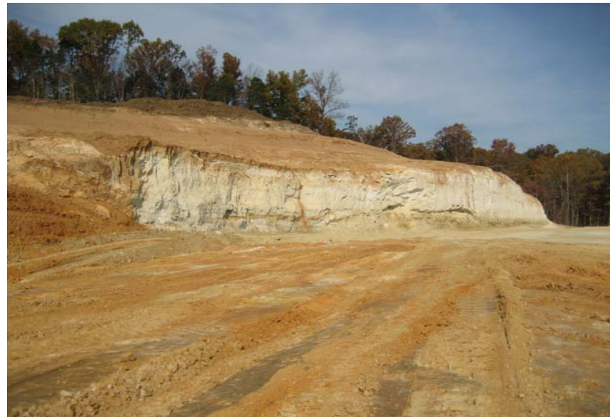
West slope and sandstone vertical wall.
