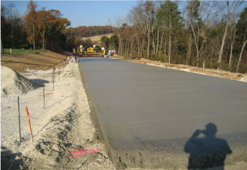
New main entrance roadway paving
