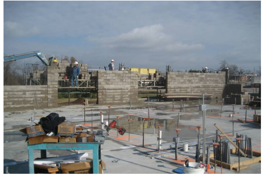
Work on north exterior load bearing wall at the office/administration area
