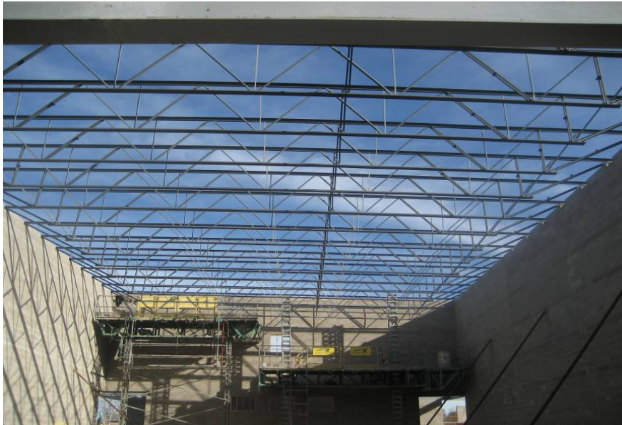
Gym long span bar joist installed with X-briding in place
