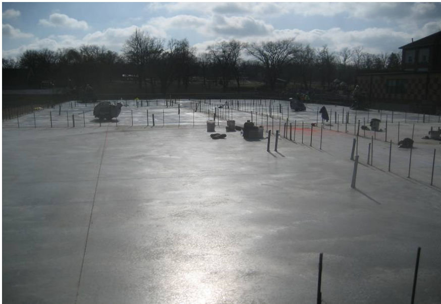
Classroom wing slab on grade poured and finished
