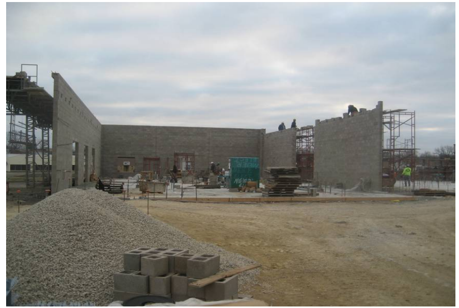
Load bearing walls of office/administration area completed
