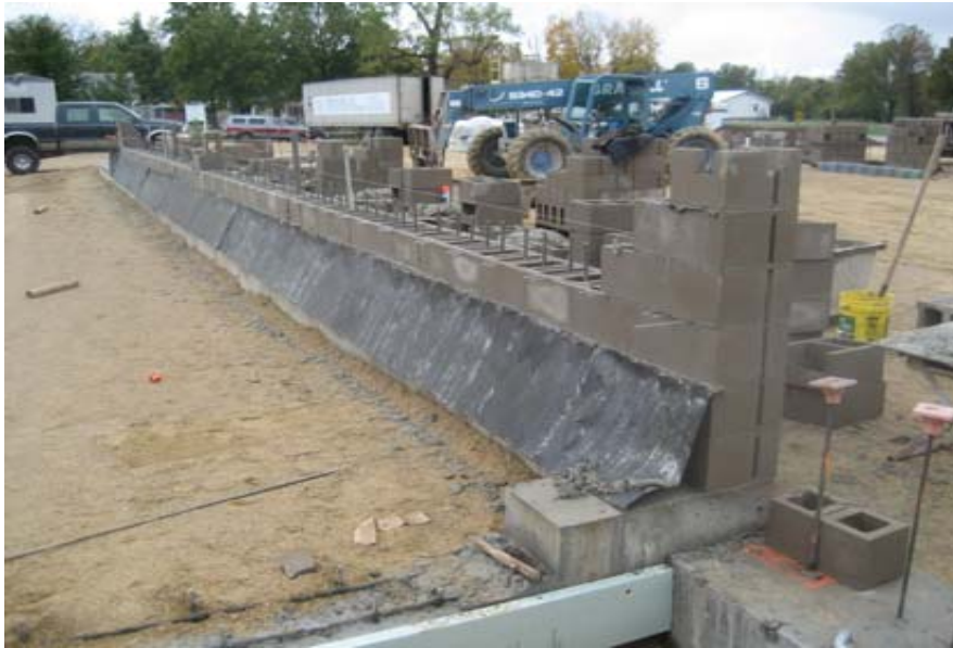
Oct. 15th - South gym wall construction
