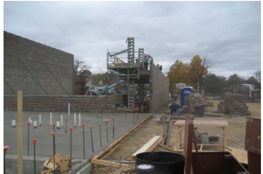
Oct. 28th - Gym wall progress
