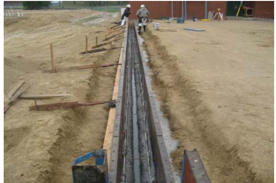
Foundation walls in gym and classroom area
