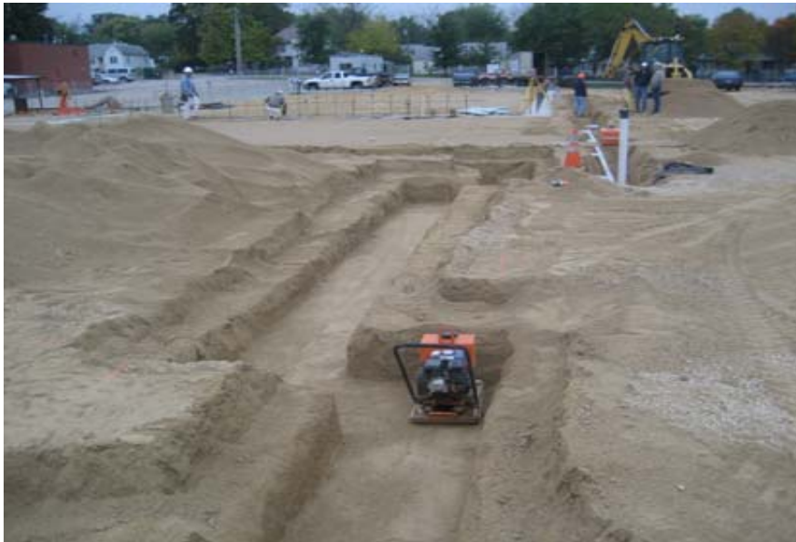
Footing dug and prepped for rebar installation
