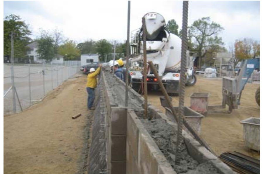
Oct. 16th - Grouting south gym wall
