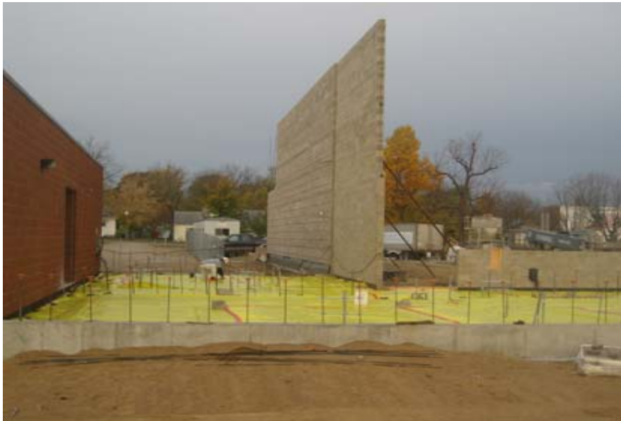
Oct. 26th - South gym wall complete
