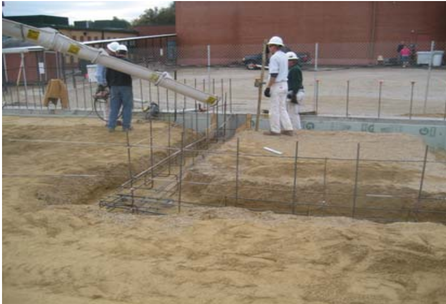
Pouring interior footing in gym
