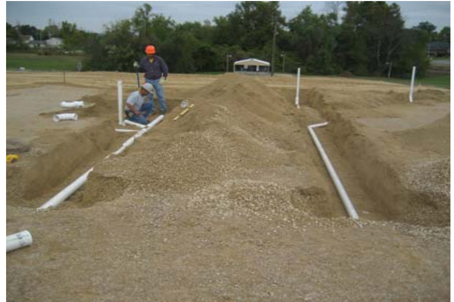
Plumbing ground rough in
