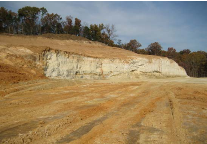
West sandstone shear wall with grading near complete.
