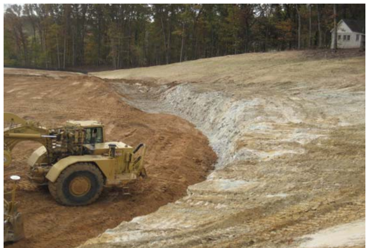
Rock removed from baseball field and replaced with clean dirt.
