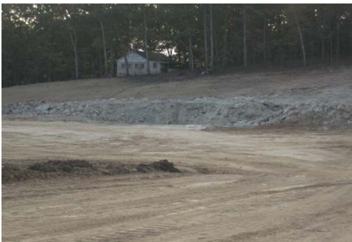
Limestone rock that has been drilled and shot from baseball field.
