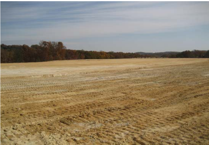
Building pad finish trimmed and proof rolled ready for building contractor.
