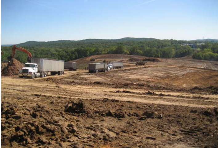
Ground tree mulch being hauled off site to a mulch recycling center to be used by landscape contractors.
