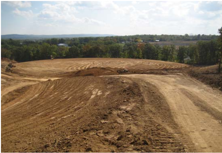
Baseball field trimmed with excess dirt piled to be hauled off.
