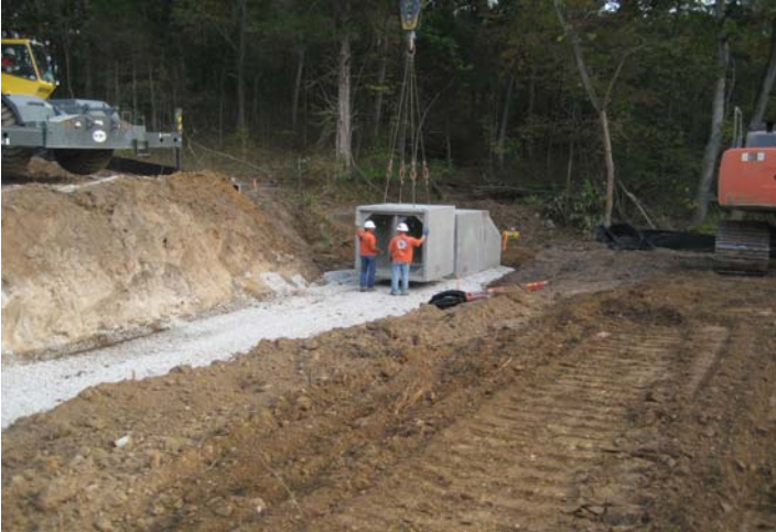
Starting to set 5' X 5' box culvert in main roadway.
