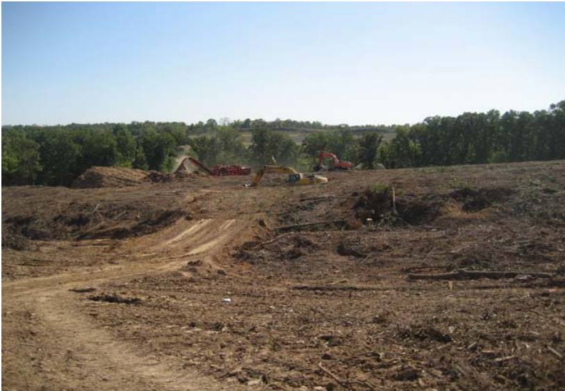
Day 8: Sept. 26th, timber cleared and chipped.
