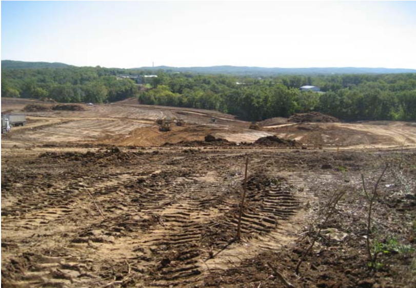
Day 11: Sept 30th, Cut fill operations at baseball field.
