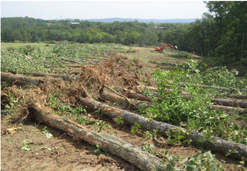
Day 1: Sept. 18th, started clearing timber.
