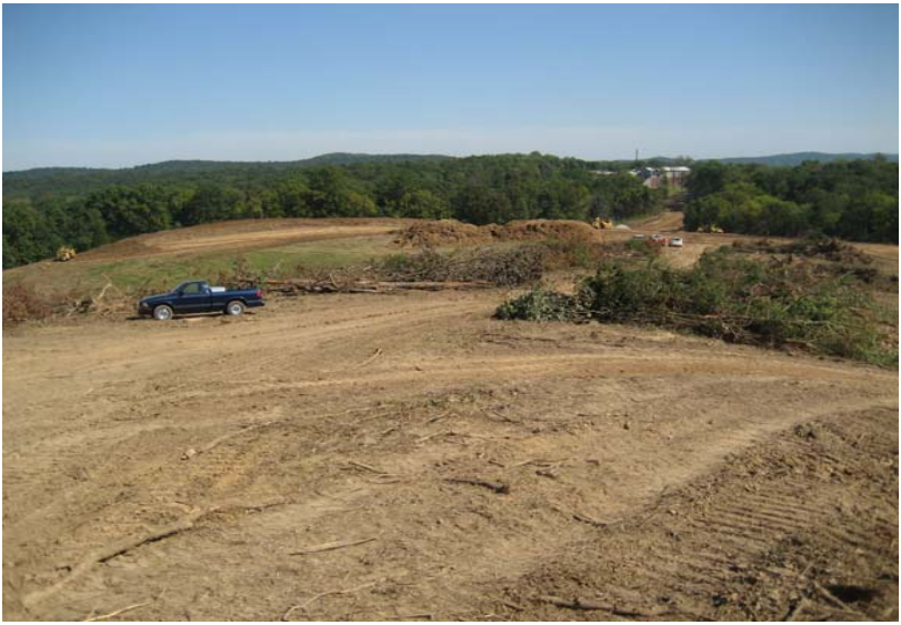
Day 7: Sept. 25th, East portion of site cleared and timber chipped.
